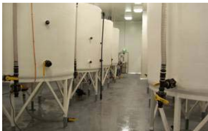
CollTech's purpose built manufacturing facility in Collie, Western Australia
